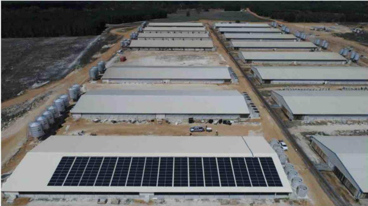
Part of stage 1 solar at Westport. Photo Supplied.
